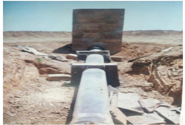
TIJO WATER PROJECT
