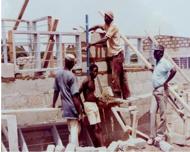
Aliu with his construction crew at the Nonrip project
