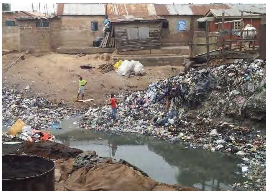
Figure 1.1: A waste-clogged drain within the Amanfrom community.
