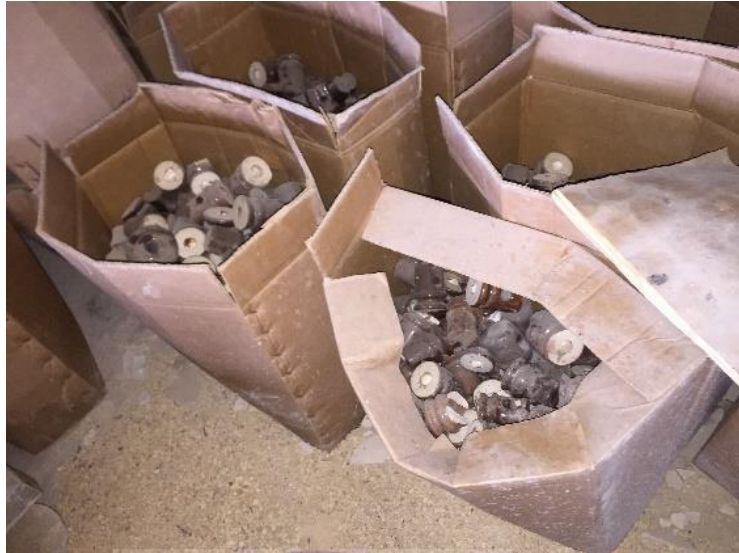
Fig 2: Sample of Electrical insulators found in the factory
