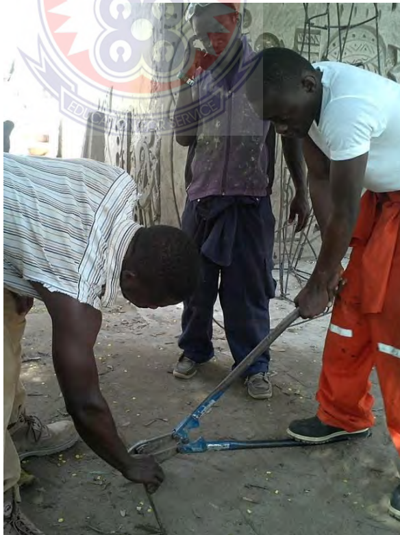
Figure 5.11(C): Cutting of iron rods
