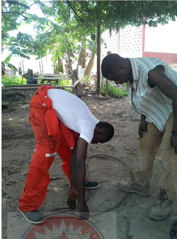
Figure 5.11(D): Bending of iron rod
