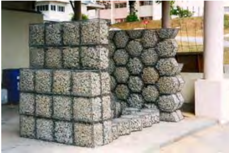
Figure 2.2: Twin Wall Construction
