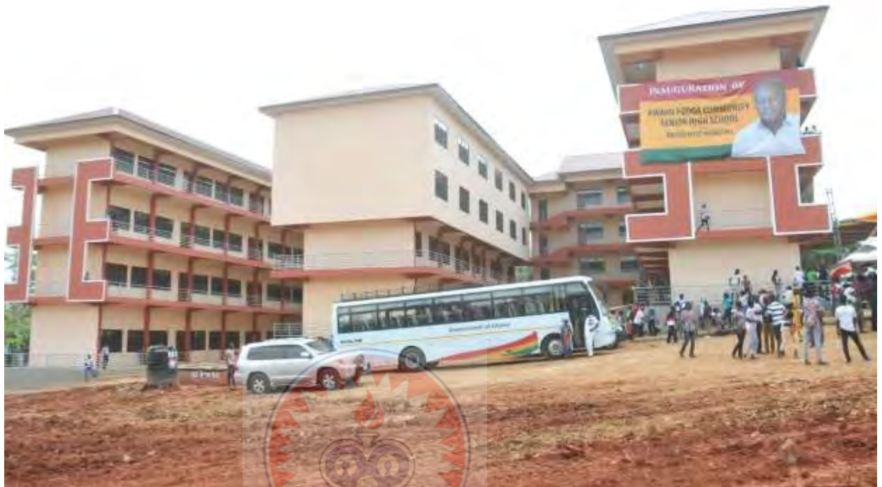
Front View of Fodoa Community Senior High School, Kwahu
