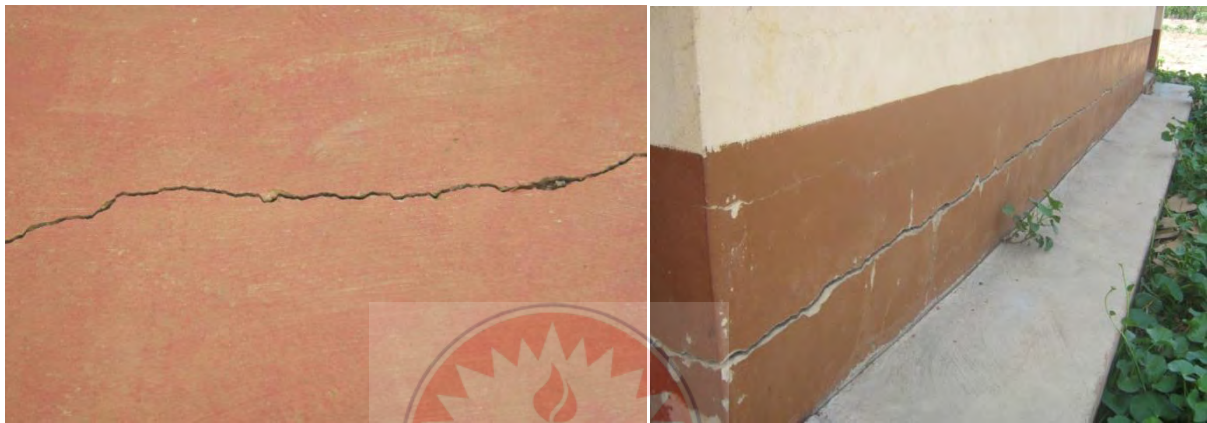
Figure 4.4: Horizontal cracks
