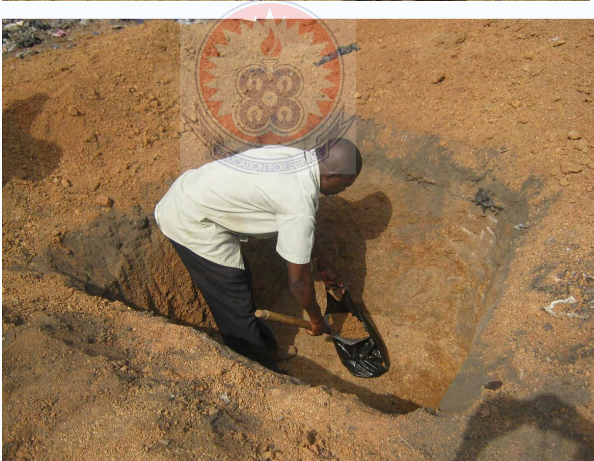
Trial pits and Dynamic Cone Penetrometer Tests at the project sites.
