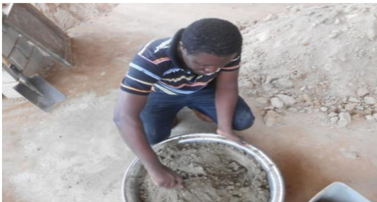
Plate 7: Mixing of mortar
