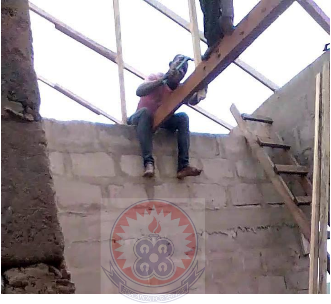
Figure 4.5: Carpenters Positioning roofing members at the top at Gomoa - Abrekum
