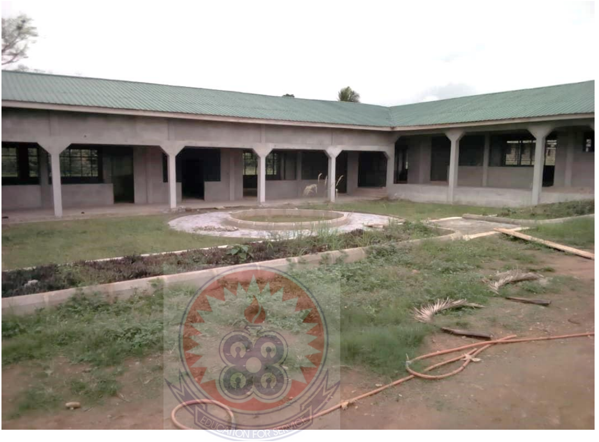
Figure 4.4: Shows a bushy site whilst workers work on internal finishing's.
