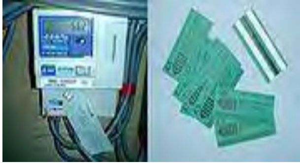
Figure 2.2: A magnetic/token prepayment system Source: Edison Electric Institute (2016).
