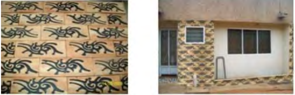
Figure 7 - Embossed Anieden Slices on a Building designed by Henrietta Barfi Mensah & Co
