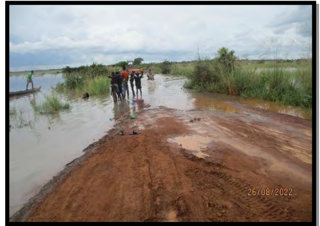
Major Road Submerged
