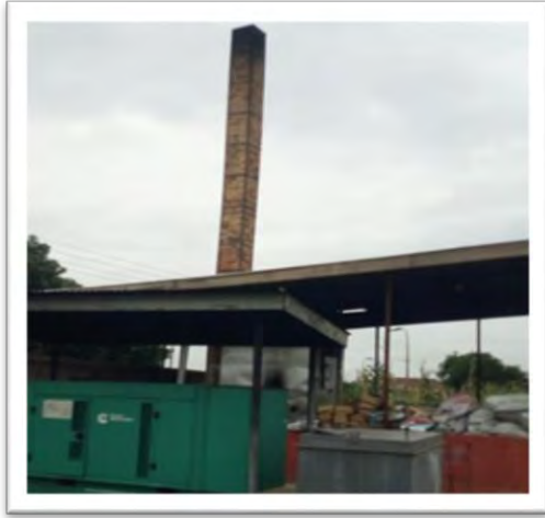
(a) Incinerator at Manhyia hospital
