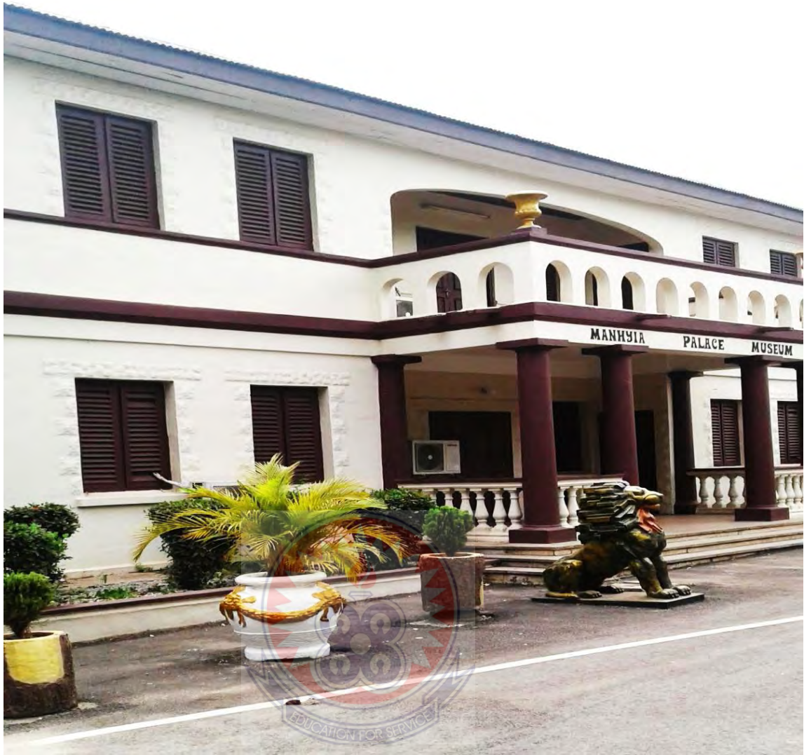
Figure 50: The Front view of Manhyia Palace Museum (Source: The Researcher, 2019).
