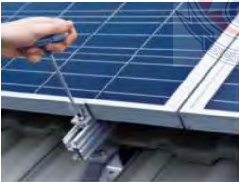
Figure 4.25: use of end clamps
