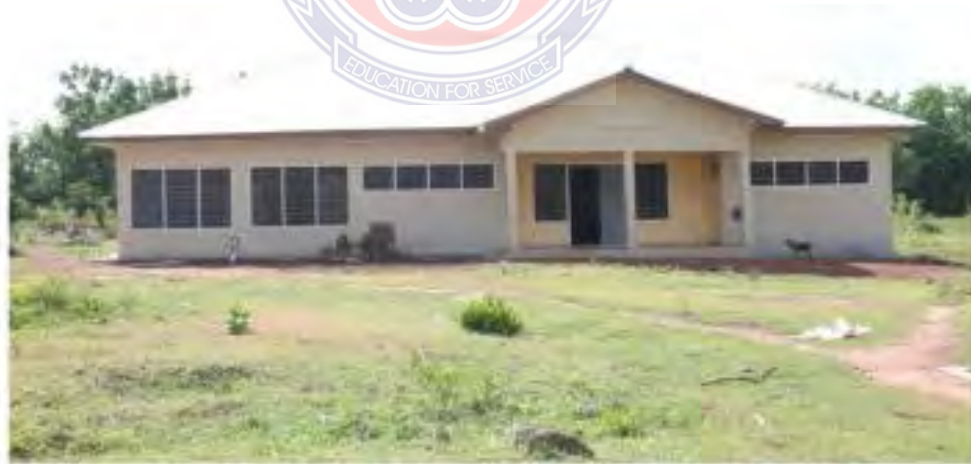
Figure 4.24: Typical roof appropriate for solar PV installation
