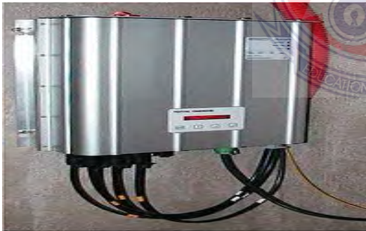
Figure 2.9: Inverter for grid connected PV
