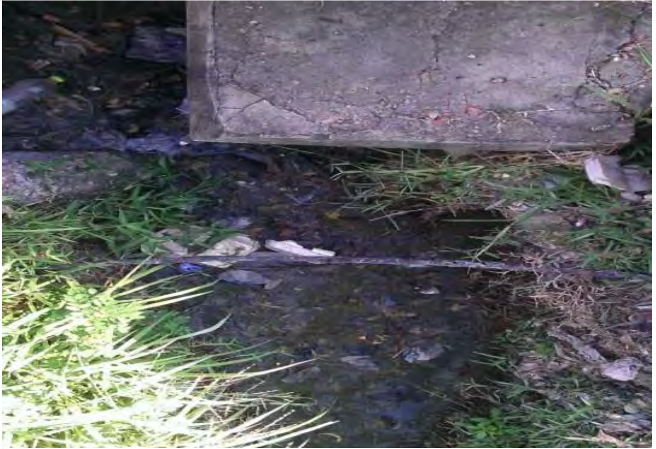
The drainage outlet from the students' hall (Winneba Campus)
