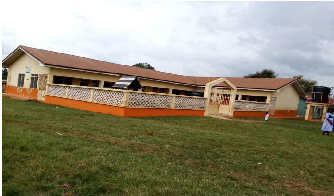
Figure 7: Front elevation of one of the preschool buildings (private)
