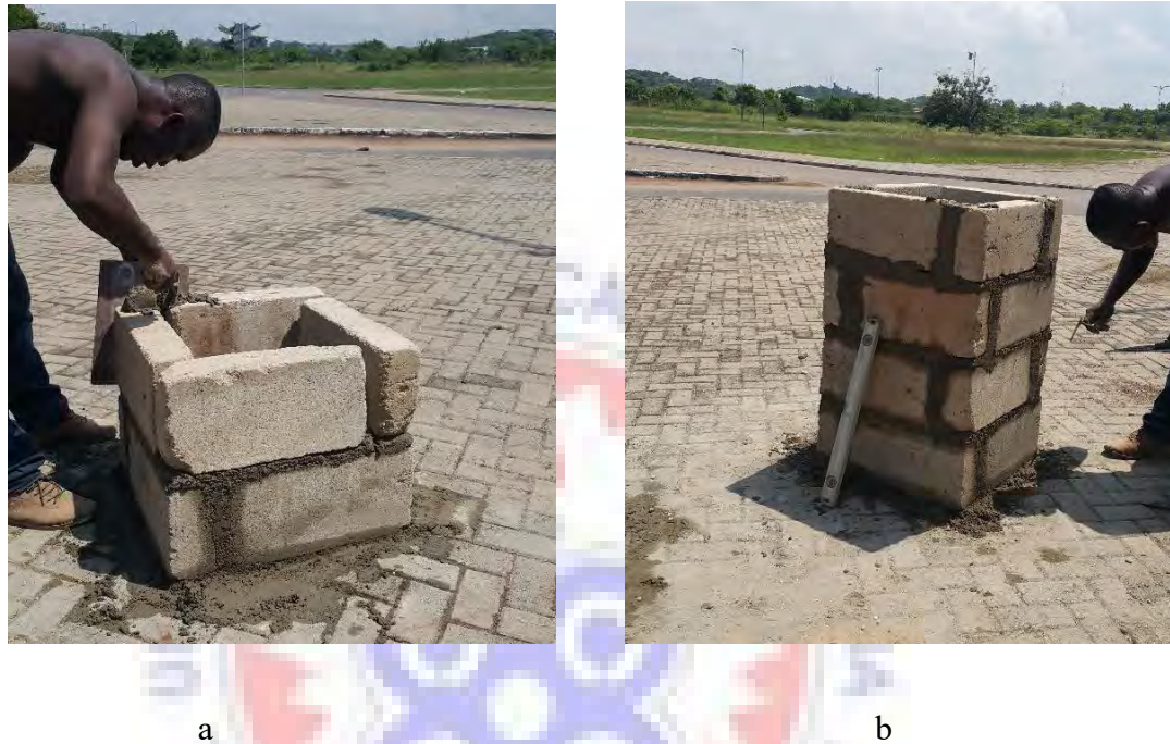
Figure 82: Block Laying
