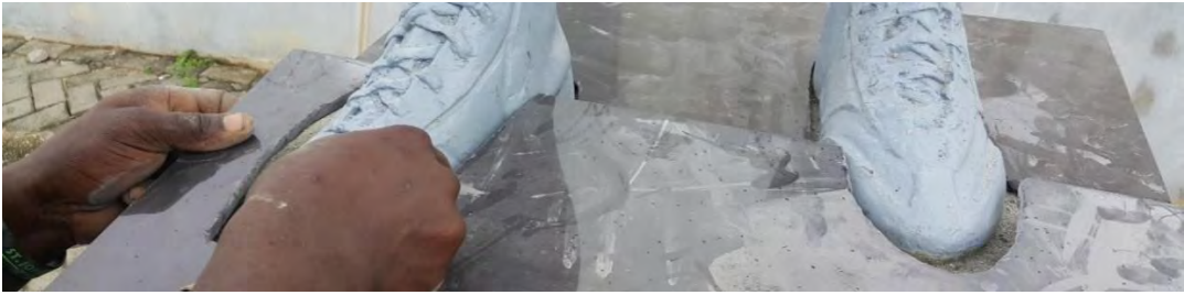
Figure 92: Tiles Joined Together
