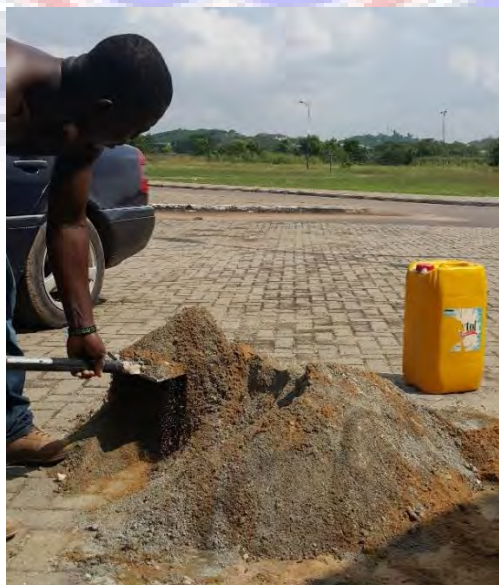
Figure 79: Mixing Sand and Cement
