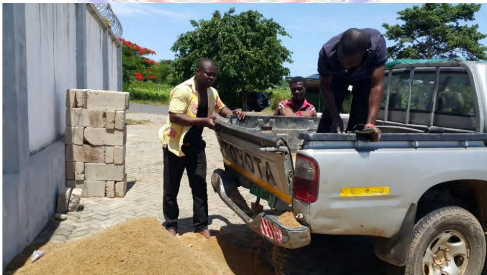
Figure 77: Sand and Blocks Conveyed
