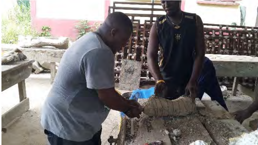
Figure 45: Binding Wire being used to Tighten the Mould
