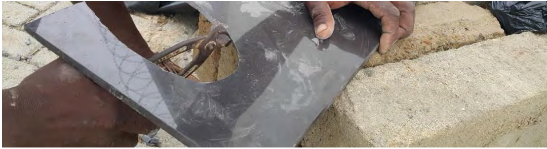
Figure 90: Cutting the Tile
