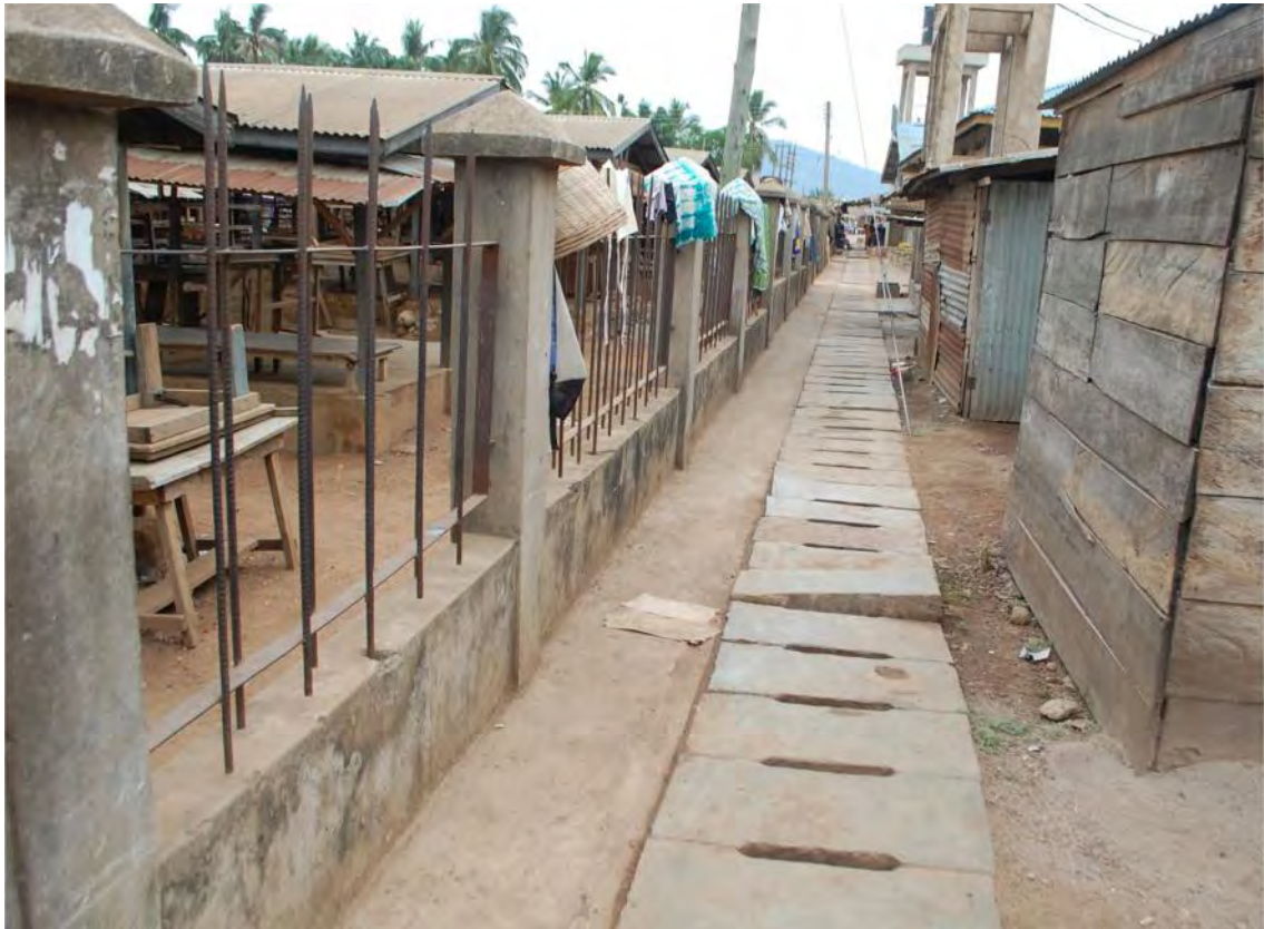
Figure 4.1: Covered drain behind chop bars and part of the fence around the market
