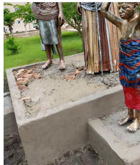
Figure 31 Complete Casting/Concreting of Pedestal
