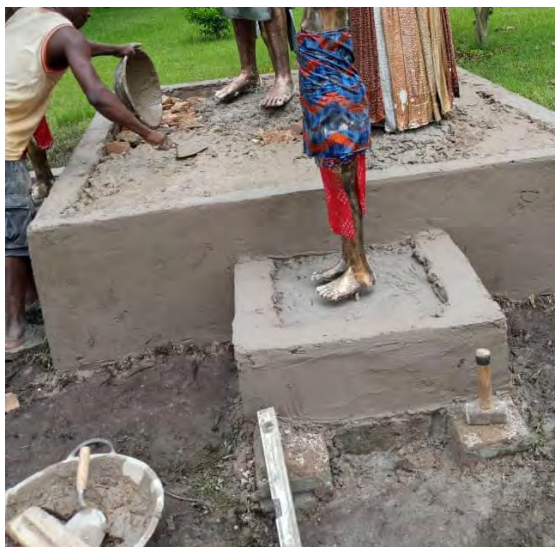
Figure 31 Complete Casting/Concreting of Pedestal
