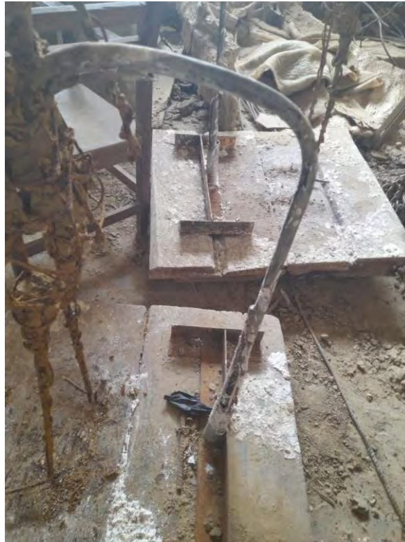
Figure 10: Armature supported with Back iron as Reinforcement (Source: Fieldwork, 2024).
