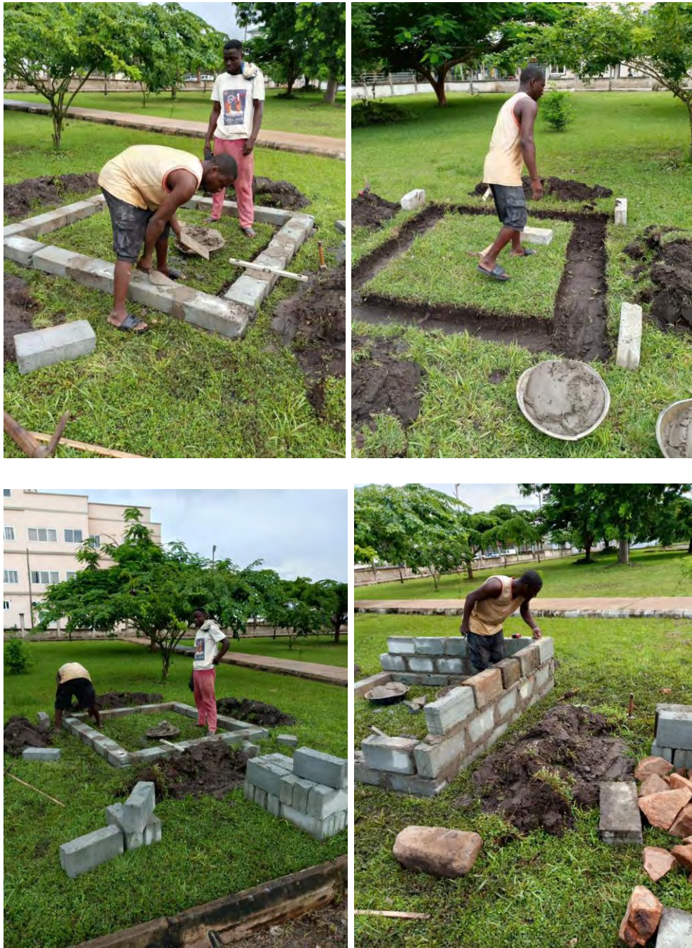
Figure 28: Laying of Blocks of the Pedestal (Source: Fieldwork, 2024).
