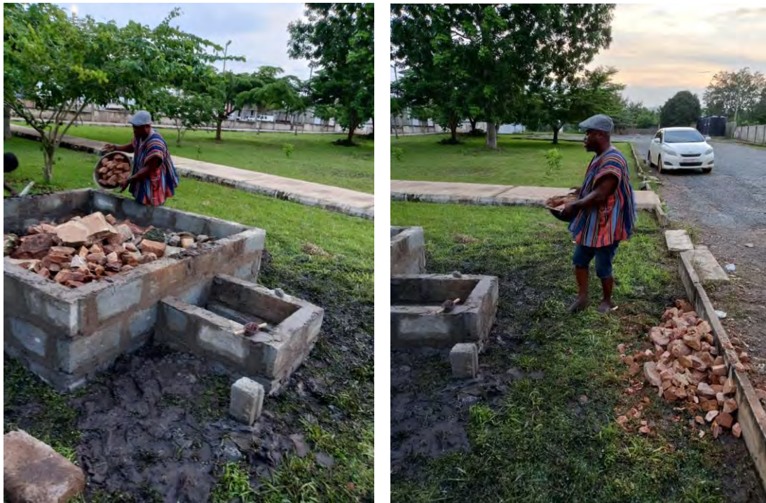
Figure 29 Filling of the Pedestal with Stones (Source: Fieldwork, 2024).
