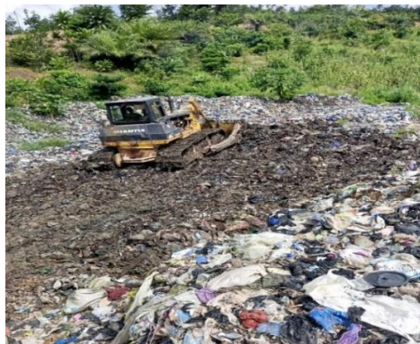
Figure 2. Compacting of waste at the final disposal site in Asankrangwa
