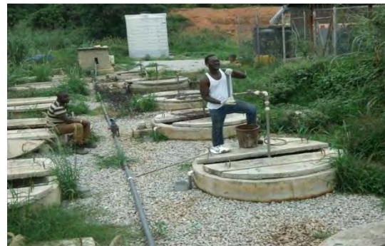
Fig. 2.4 Worker Measuring the Quantity of Oxygen in a Bio-Digester
