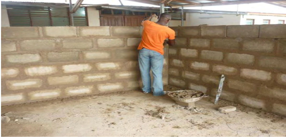
Fig 3.2: Sandcrete block wall
