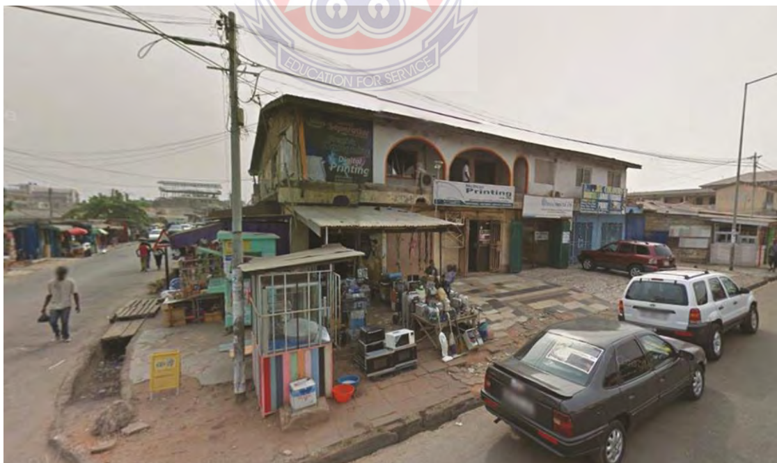
Figure 14. A house engaged in printing business, Accra New Town (Source: field data, 2019)
