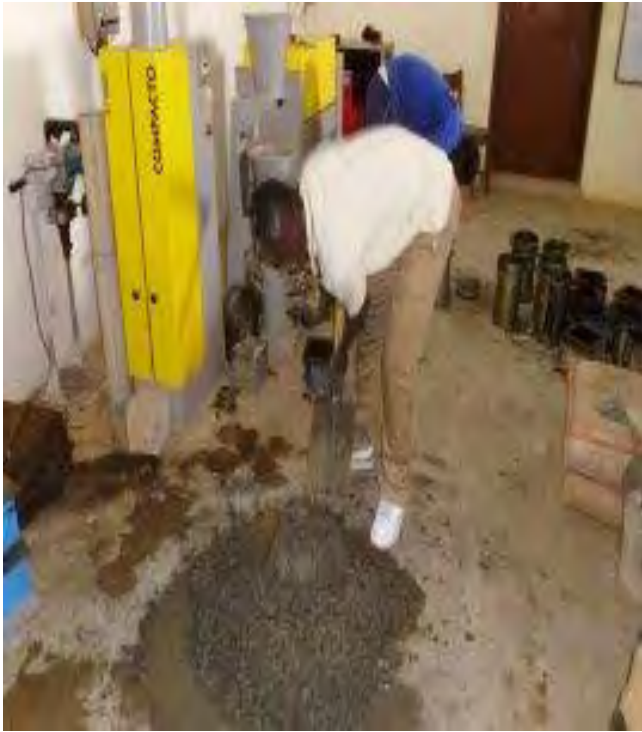
A 5 Mixing of Concrete by Hand
