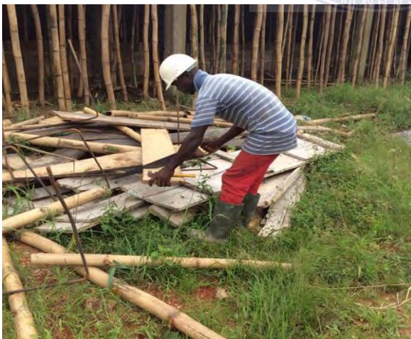
Figure 4.3: A construction worker wearing a helmet and wellington boots for protection.
