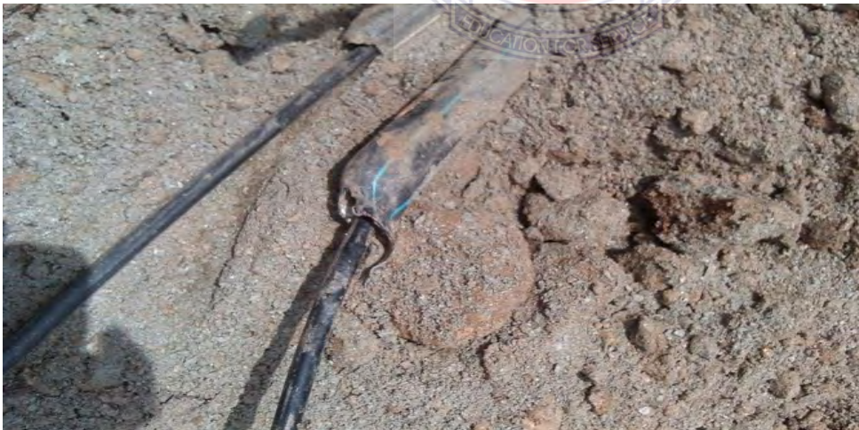
Figure 7: Duct installation method (TIGO)
