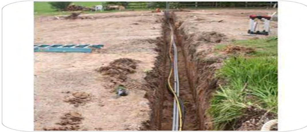
Figure 8: Direct buried installation method (used by MTN)
