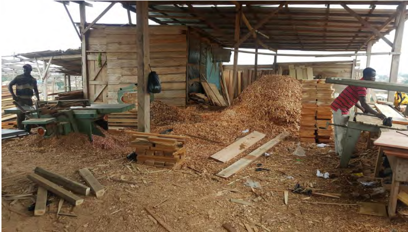
Plate 2.3 woodwork machine operators with no safety gadgets on working in a very unkept machine shop.
