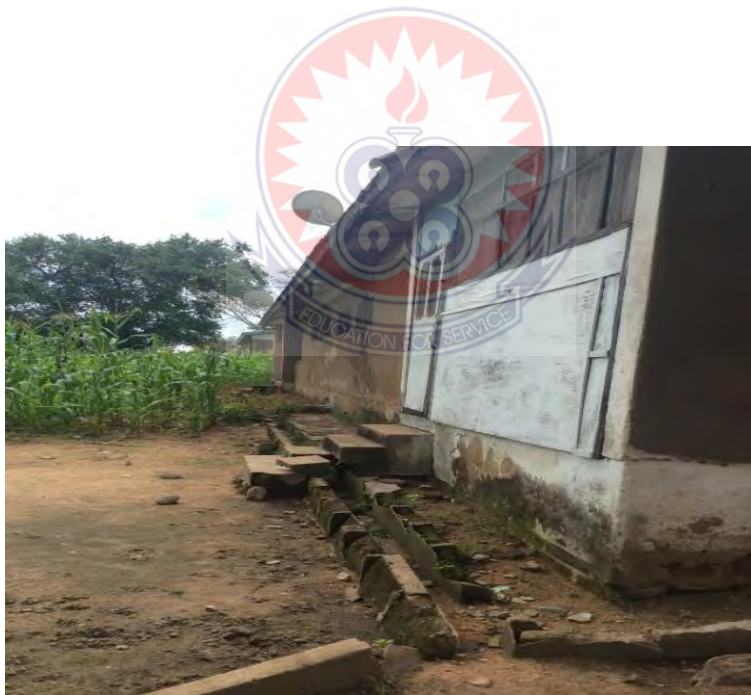
Weak substructure
