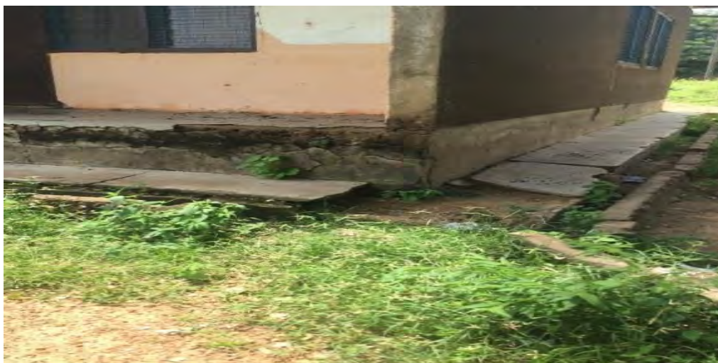
Figure 4.4: Weak foundation/substructure
