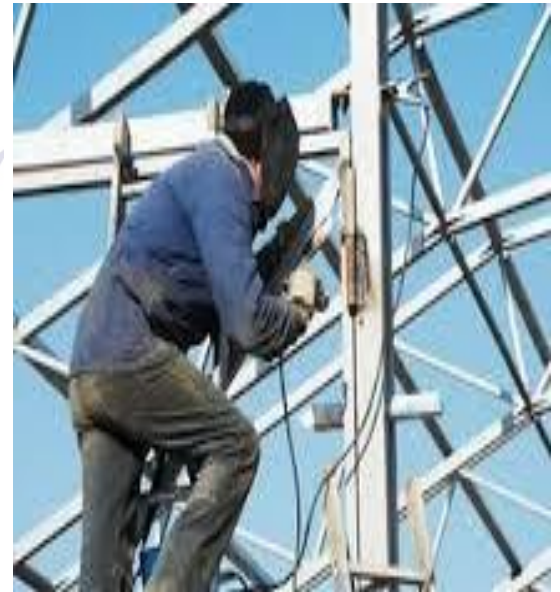
Plate 11:- apprentice working on site
