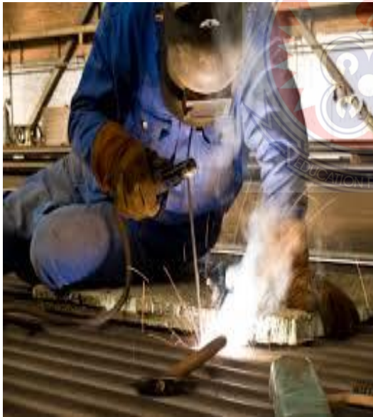
Plate 10:- apprentice working on site
