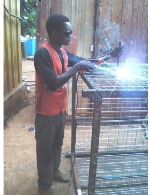
Plate 5:- apprentice welding a cage
