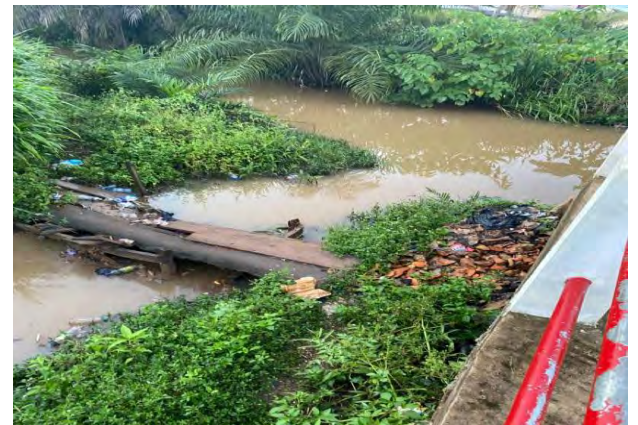
Aftermath of flood, Liberty, Akim Oda.
