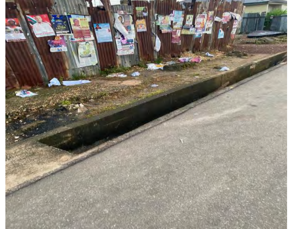
Installed drainage at Jamaica, Akim Oda.
