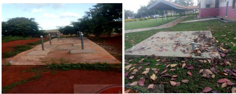
Figure 5.6: Mampong Hospital Sewer (Source: Field Data, 2020)
