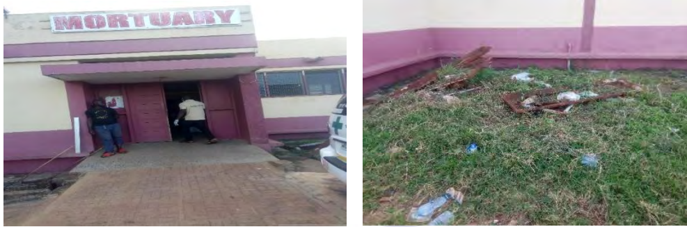
Figure 5.4: Mampong Hospital Mortuary
