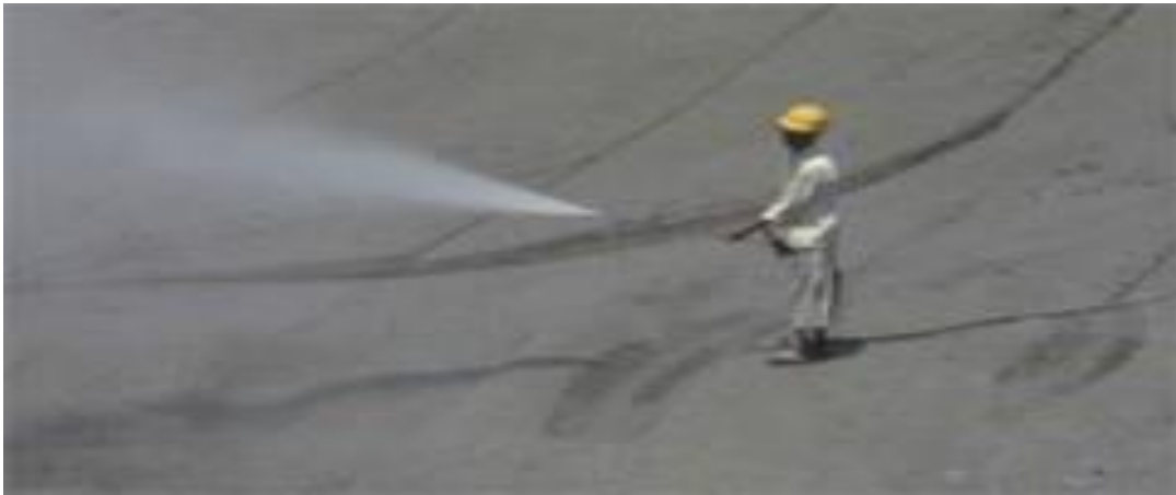
Figure 2. 4 : Mist curing of freshly placed concrete
