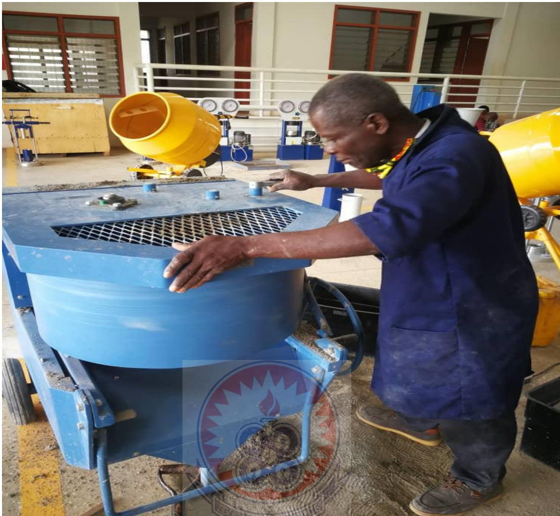
Figure3. 5 mixing of the mortar
