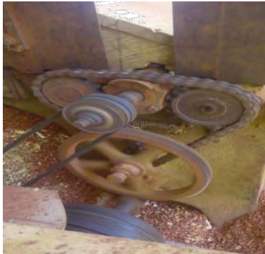
Figure 4.16: Circular saw without guard for belt and pulleys
