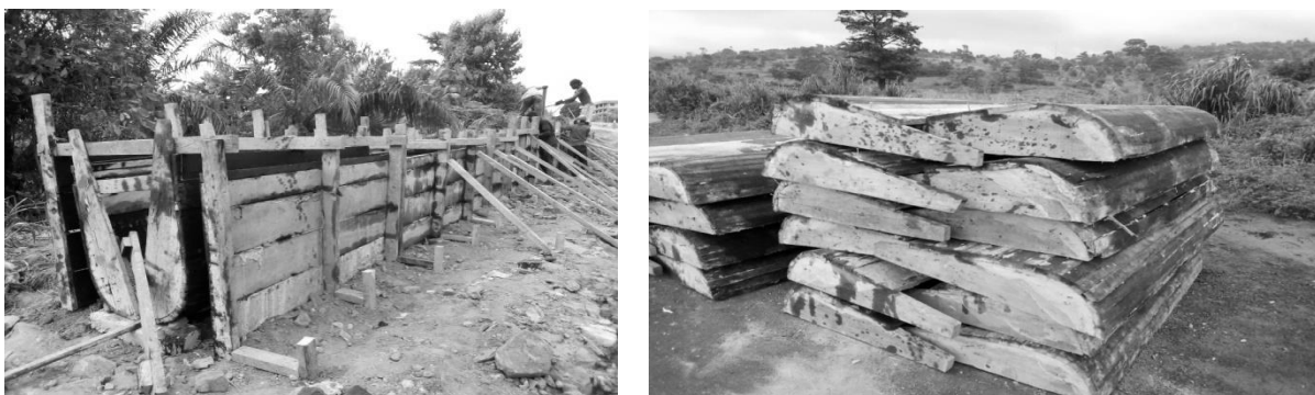
Figure 2. 1: Formwork for the construction of drains (Site Visit).
