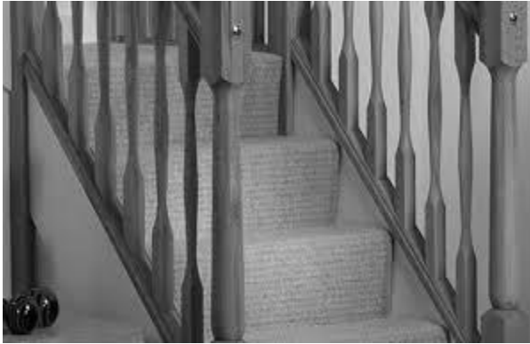
(a) Wooden staircase
