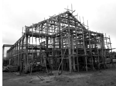
(d) Scaffolds made of timber
