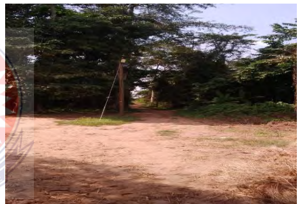
End of Extension of Lighting System
