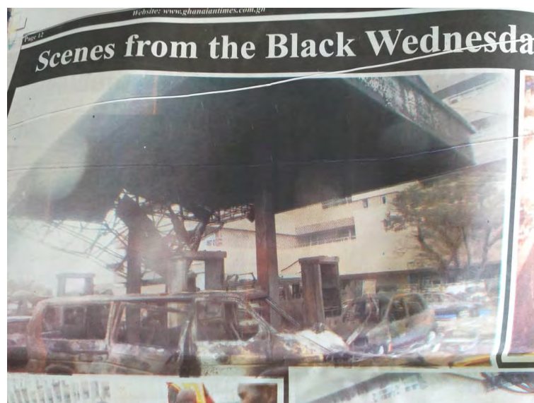
Figure 4.3: Photograph (Ghanaian Times, 6 th June, 2015) from the Newspapers Showing Destruction to Property (p.12)
