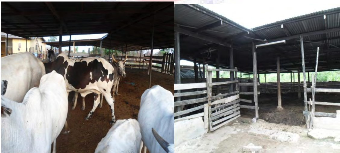
Plate 3.3d: Roofed kraals with metallic and/or wooden walls.
