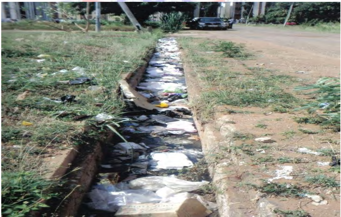
Figure 4.3: a gutter in front of a cage being filled with solid waste. February 23, 2013
