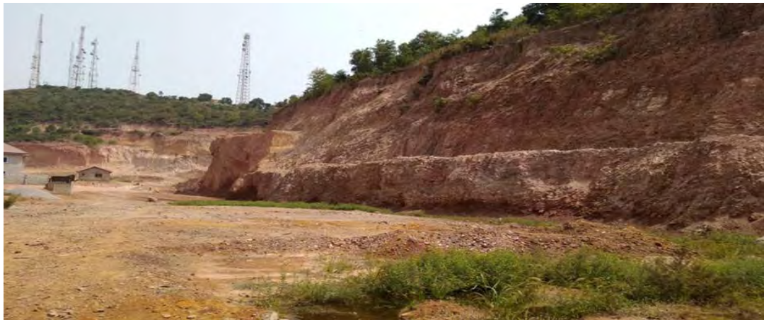
Figure 9: Showing portions of the hills that has been become steep due to quarrying and lowered portions prepared for development at Site B
