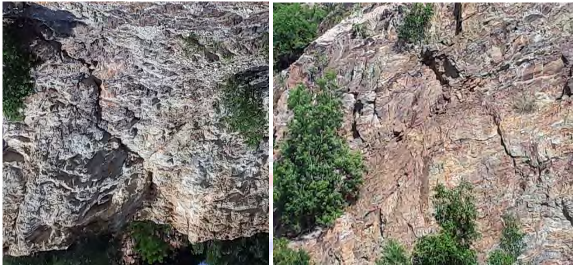
Figure 7: Showing cracks in rocks after being exposed by quarrying at Site A
