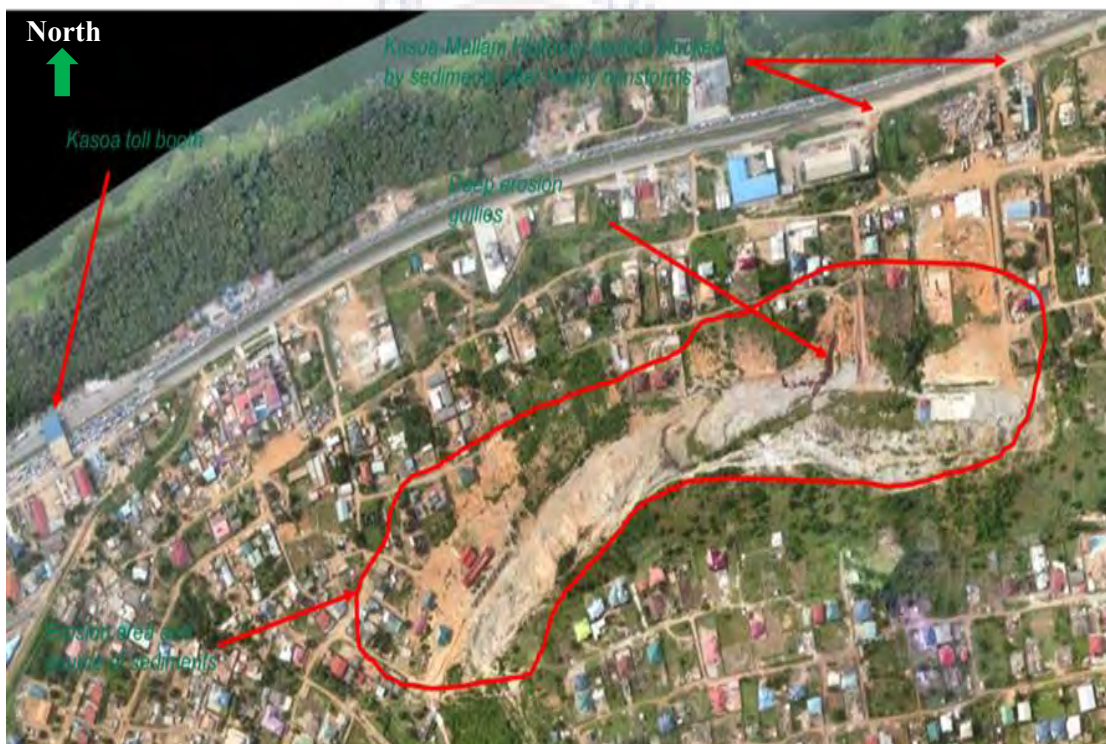
Aerial view of Akoasa Mountain problem area taken from drone.
