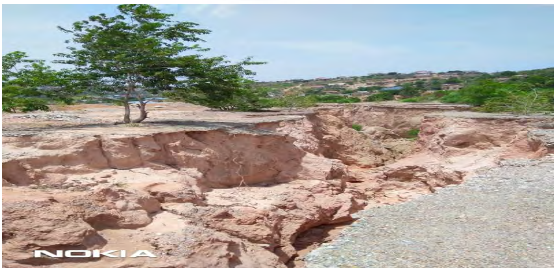
Figure 8: Showing cracks on quarried floor widened by erosion at Site A
