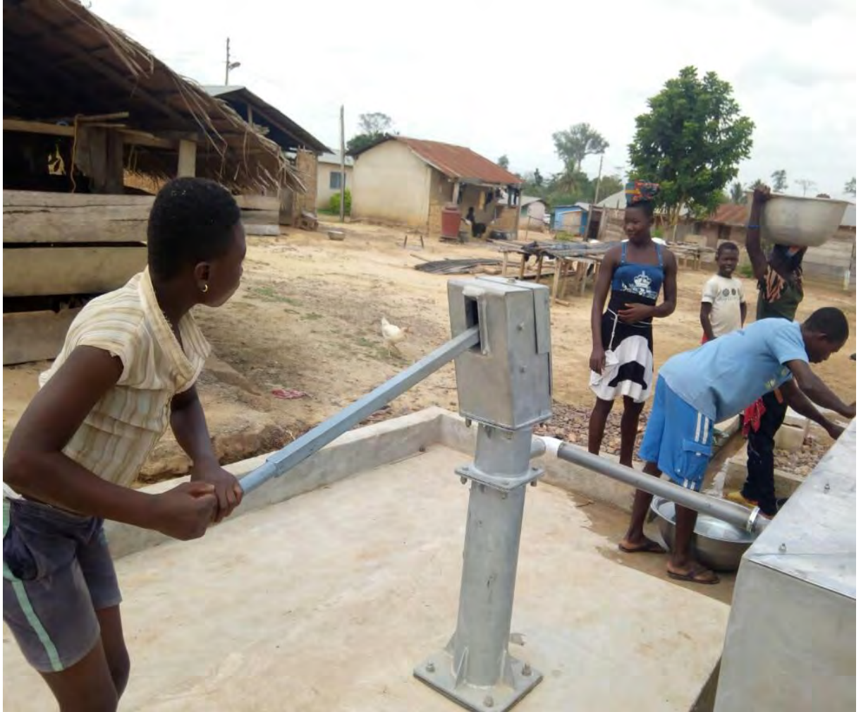
Image 4: Borehole provided by USAID and Global Communities in Aseikrom.
