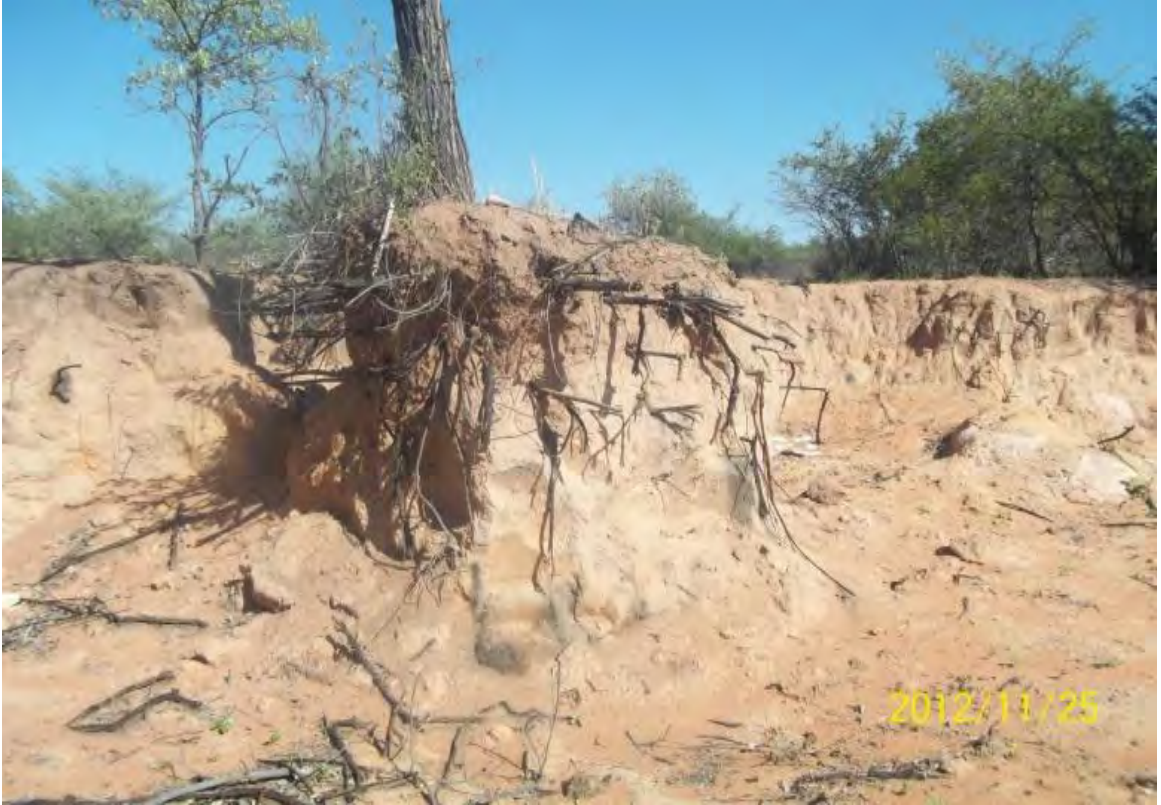
Figure 4.4 Exposed roots of a tree due to excessive sand mining at Akwadum
