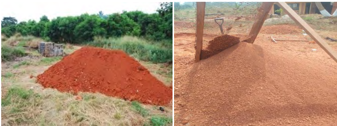
Figure 3.3: Laterite used for moulding interlocking blocks was sieved.
