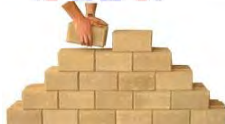
Laying of Interlocking blocks by the artisan.
