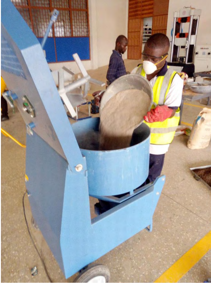
Pouring of Sand onto the Pan Mixer
