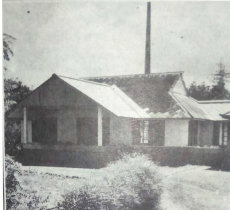
Figure 4.3. Station ZOY, The Bungalow of the first Broadcasting House in Accra (1935)
